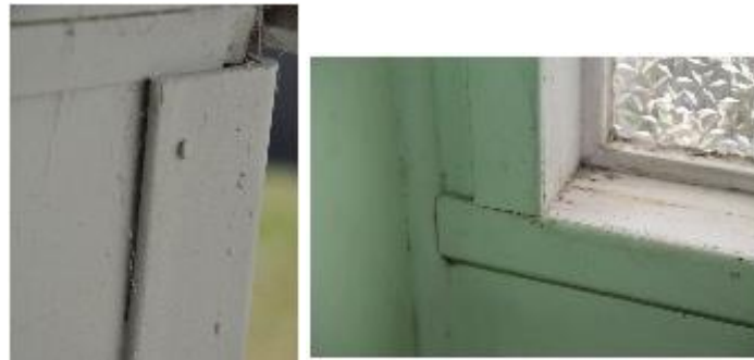
Door, Window, Cornice and Joining Strip Mouldings.
